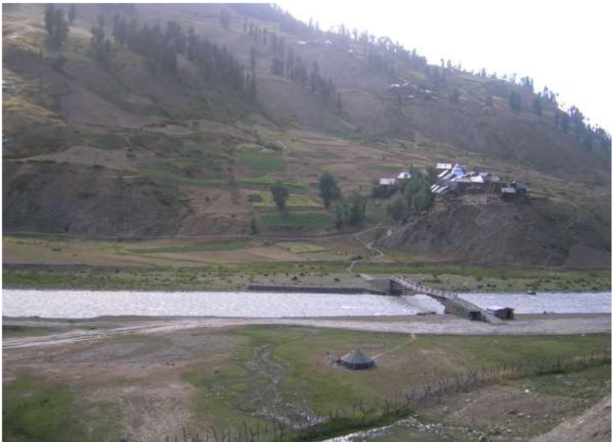
Fig.35: Bridges connecting populations across the physical barriers of streams
