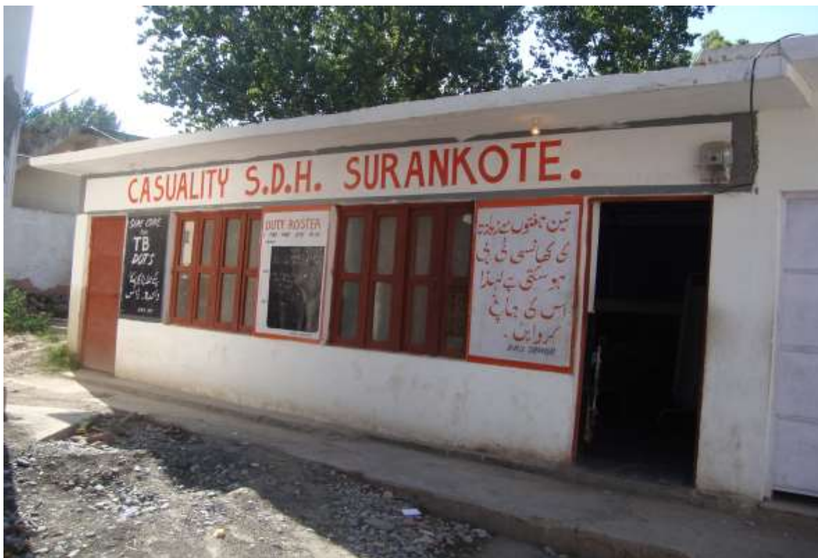
Fig. 113:Casualty block of Sub District Hospital, Surankote, Poonch District
